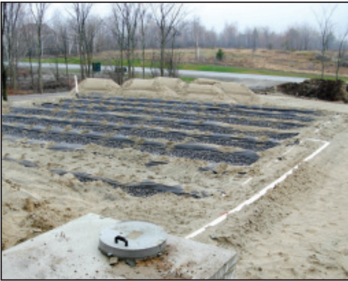
Leaching bed with perforated PVC drain pipes.
